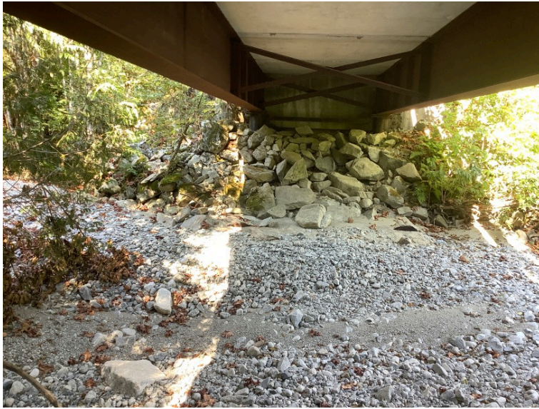
Left Bank Abutment when facing downstream
