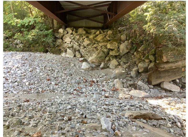
Right Bank Abutment when facing downstream
